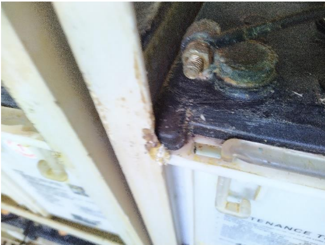
Figure 16 - Galvanic reaction.
