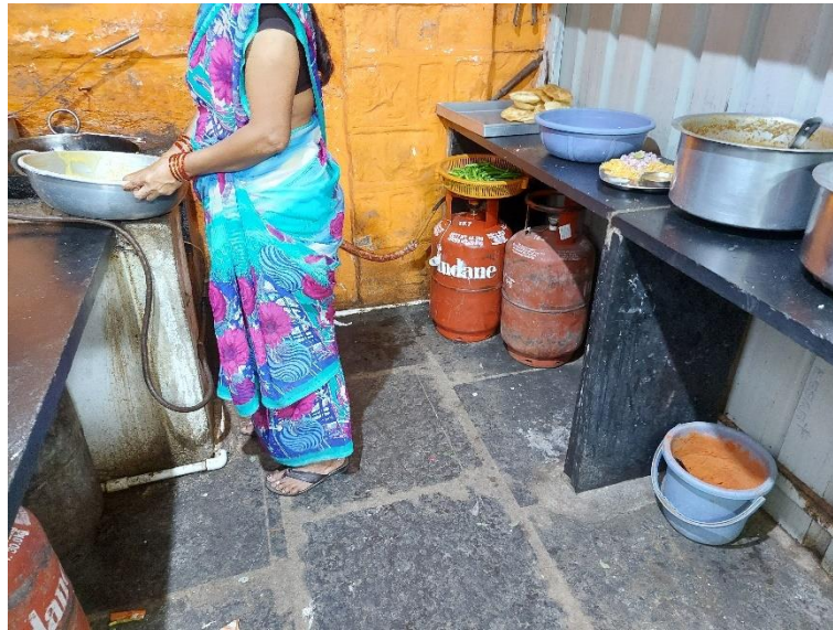
Figure 23 - Placement of LPG cylinders in wrong location.
