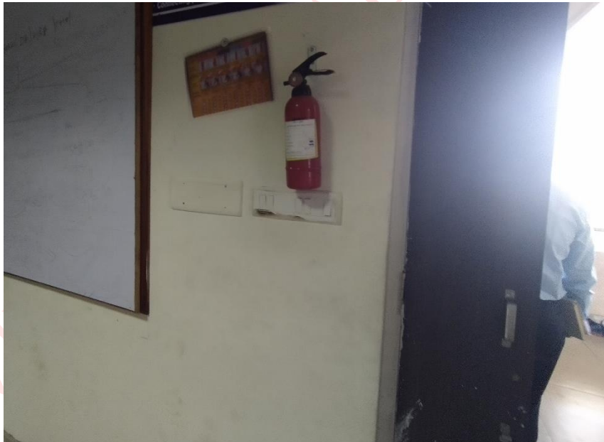
Figure 19 - No ready access to fire extinguisher.
