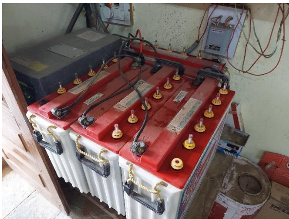
Figure 14 - Placement of battery is in danger
