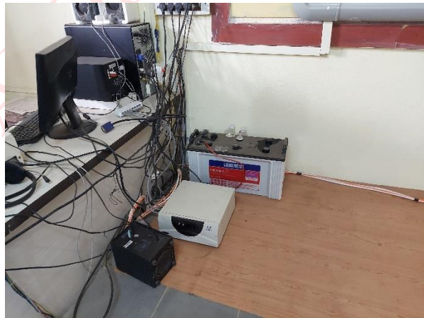
Figure 14 - Placement of battery is in danger
